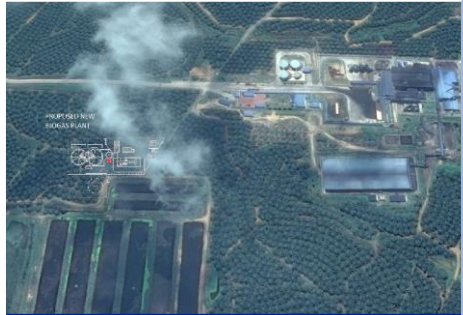
Biogas Plant at Kulai, Johor. JV with Sime Darby
